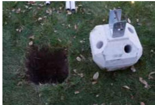
**Figure 3. Tapered Hole for Concrete Head**
