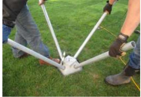
**Figure 4. Setting Pins and Leveling Pier**
